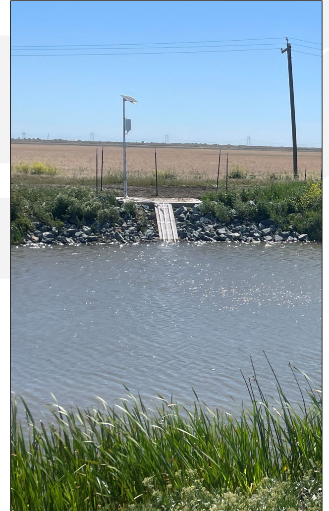
RD 2068 Main Canal – Channelmaster site
