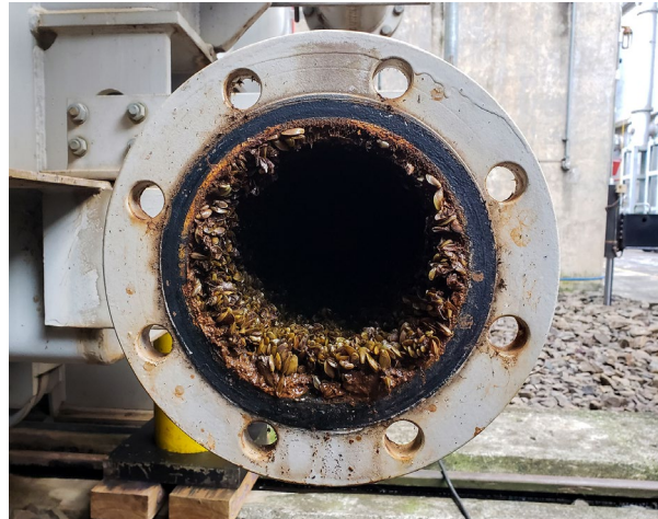
Golden mussels in pipe at hydroelectric plant in Brazil (Science.org 2021)
