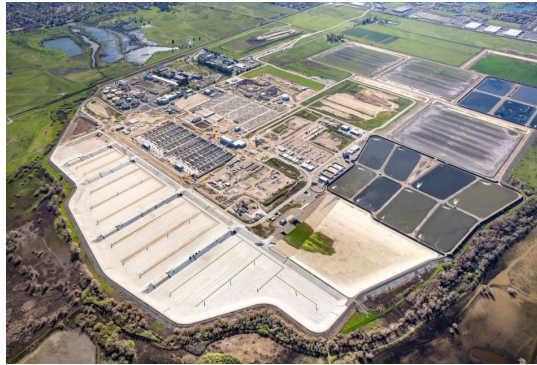
Figure 3. Sacramento Sewer District's EchoWater Resource Recovery Facility (EchoWater). This facility treats on average 135 million gallons of wastewater per day.
