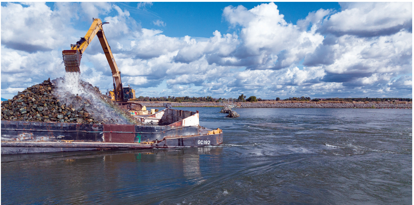
Construction crews working on removing an emergency drought salinity barrier in Contra Costa County
