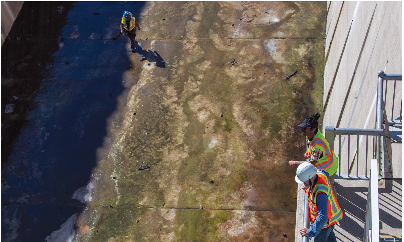
Engineers inspect the outer wall of a spillway
