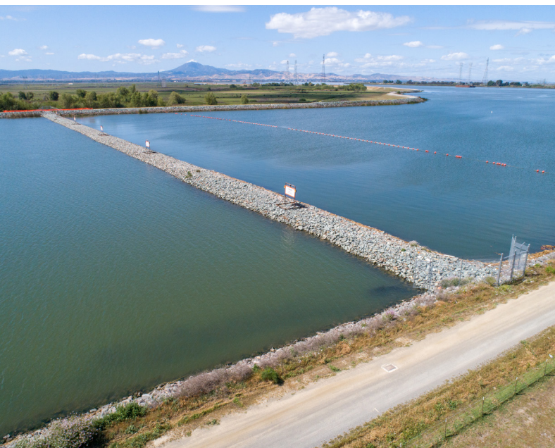
Emergency drought salinity barrier on the West False River near Oakley
