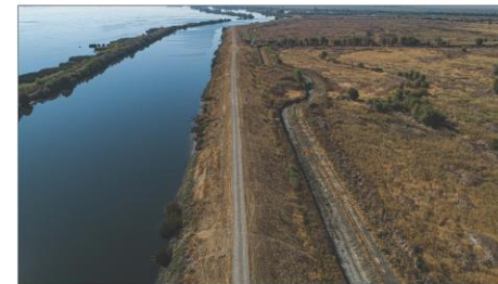
Existing levee pre-construction (will be breached)
