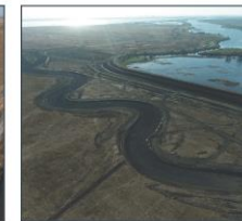
Site in progress as of October 2022 (interior channels constructed)
